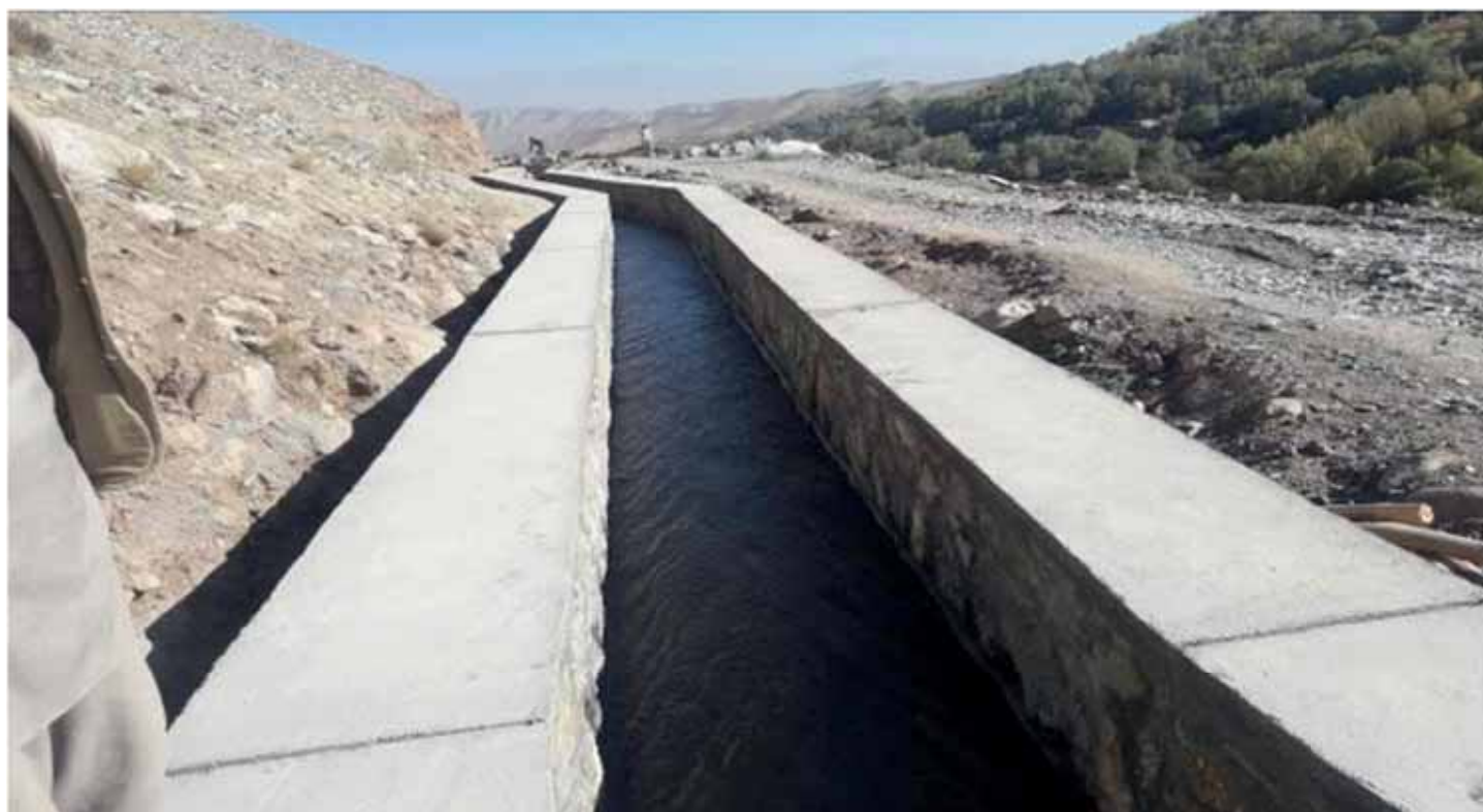
Irrigation canal constructed in Bamyan by CAWC and funded by UNHCR
